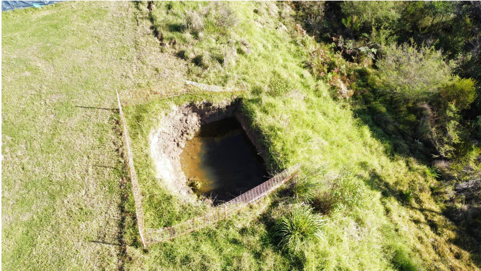
Large excavation immediately adjacent to batter with water in base
